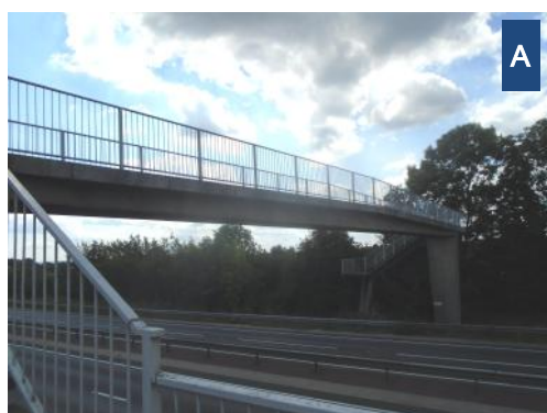
Bridge over A34
