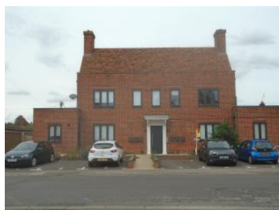
Old Saxton Arms, now apartments
